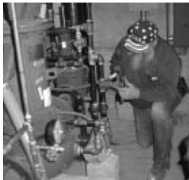
A sprinkler fitter from Superior Mechanical adjusts a tamper switch.
