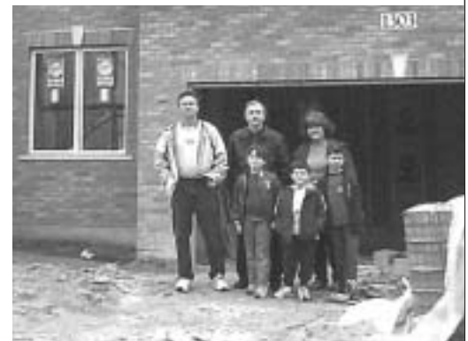
Builder Rich Laurenzana (left) with the Zibrat family in front of their new home, complete with a fire sprinkler system.
